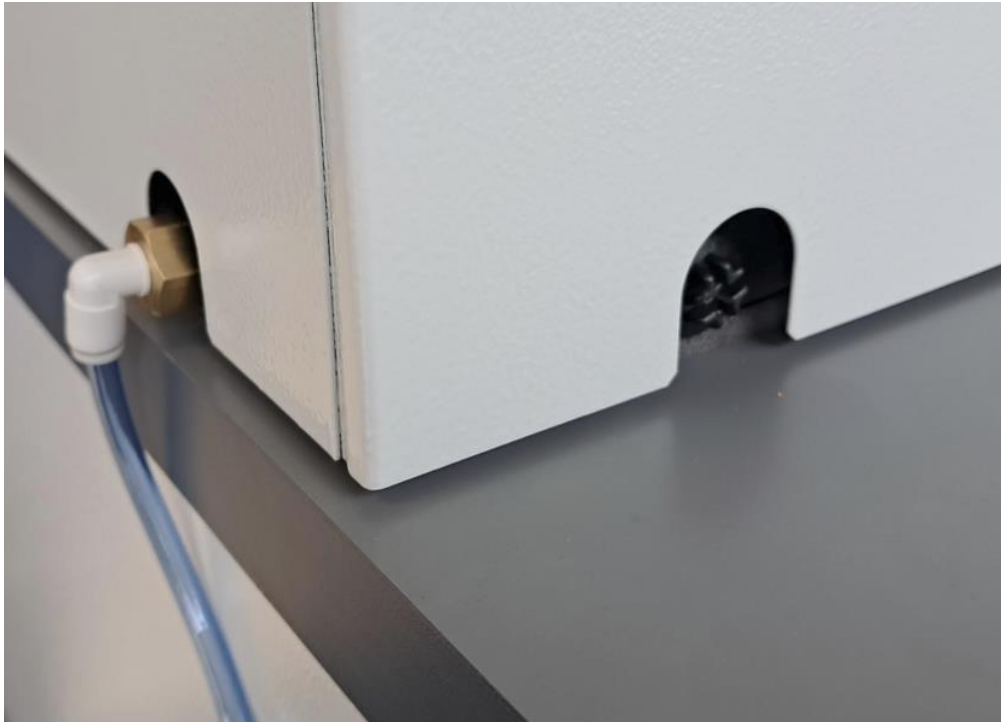
Figure 21: The condensate outlet ports on the air-conditioning unit
